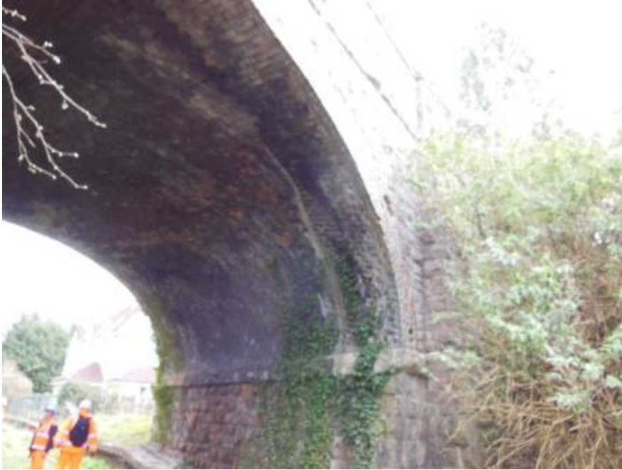
Figure 25- Arch soffit of overbridge adjacent to old Portbury Station
