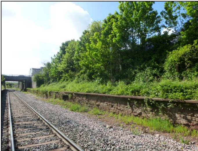
Pill Station platform – Lineside view
