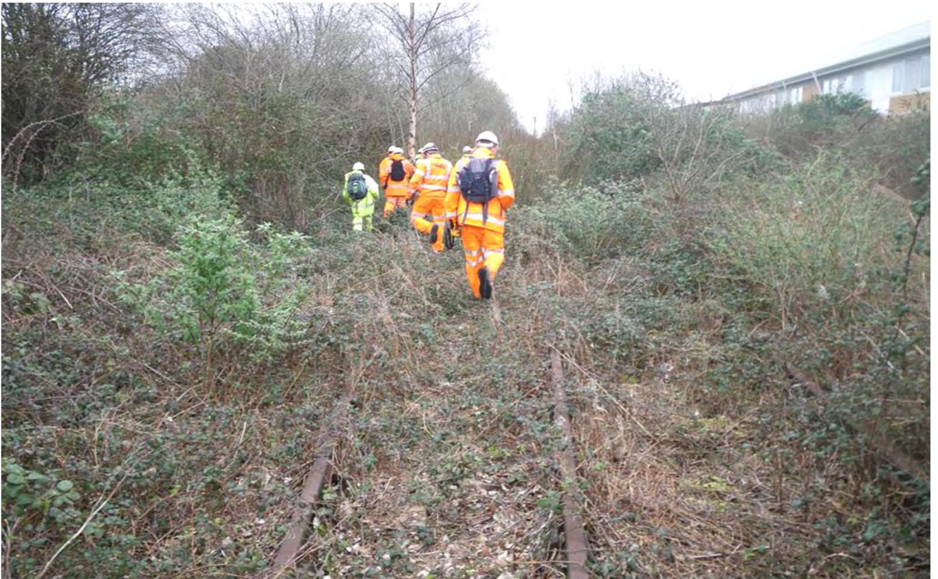
Photo 2. Facing Portbury Jcn at 129m 766y
