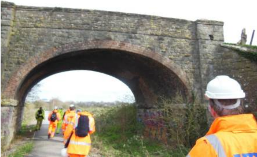
Figure 34 - Overbridge high mileage end – Marsh Lane
