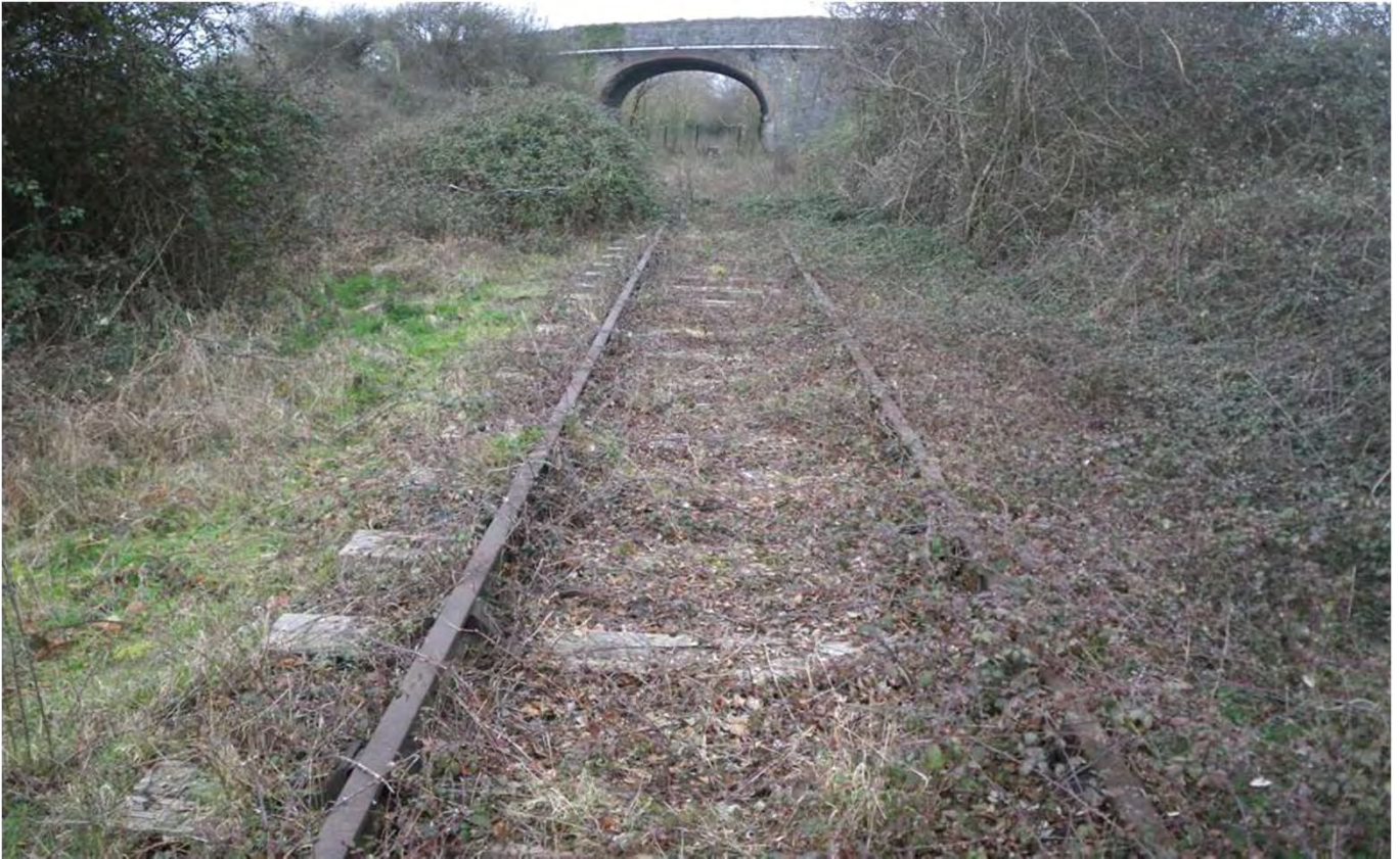
Photo 23. Facing Portishead at 128m 1168y: Sheepway Road Overbridge
