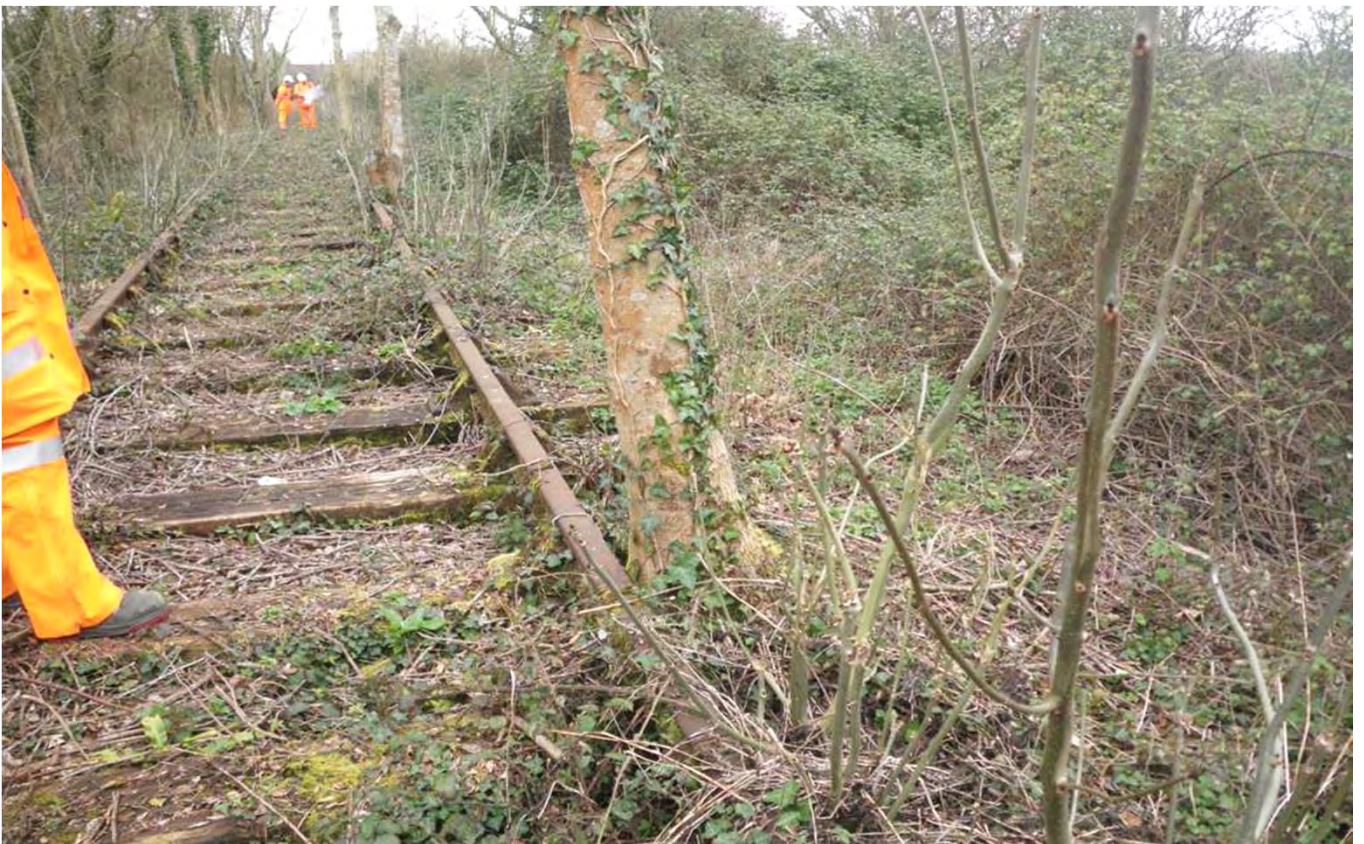
Photo 18. Facing Portbury Jcn at 128m 1450y
