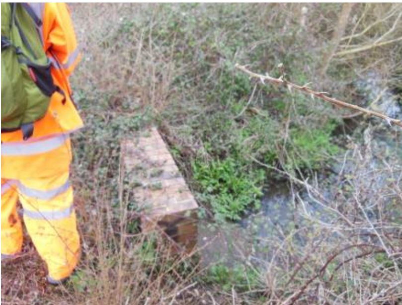
Figure 17 - Drainage channel / culvert
