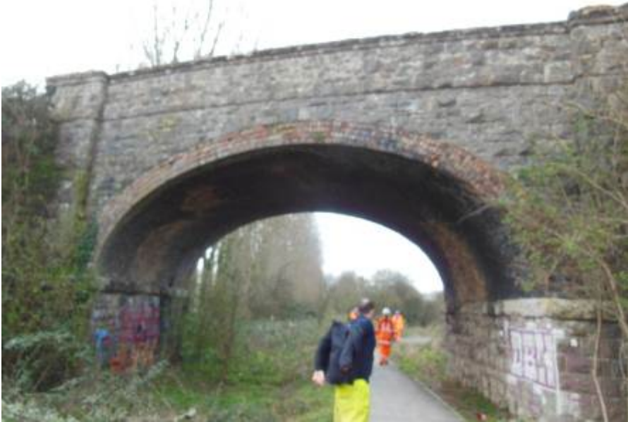
Figure 35 - Overbridge low mileage end – Marsh Lane
