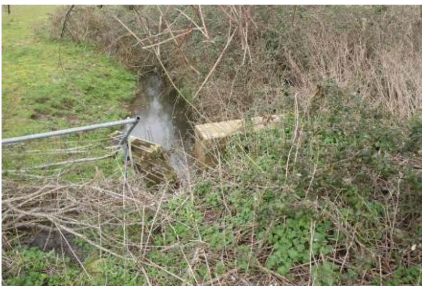
Figure 23 – View of culvert from track
