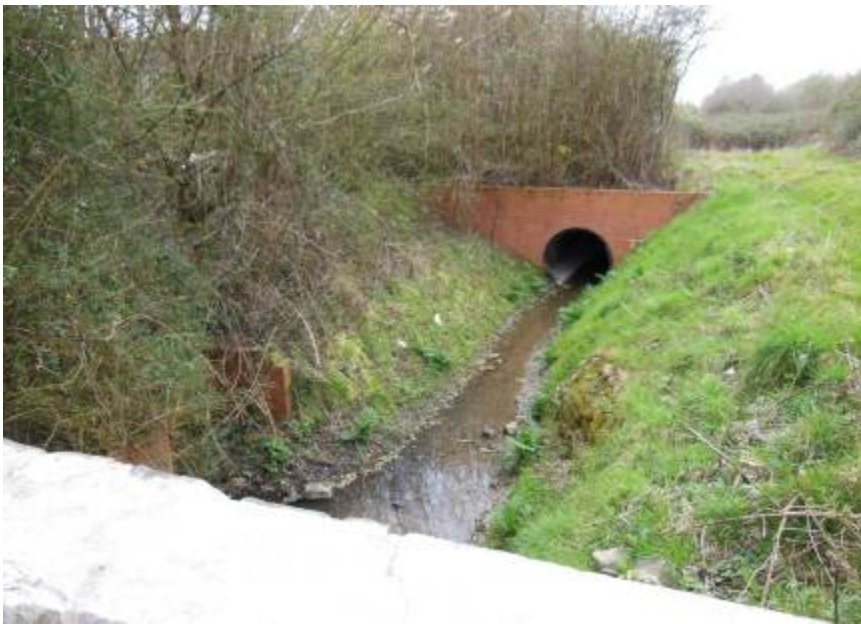
Figure 4 - Culvert lying to South of line
