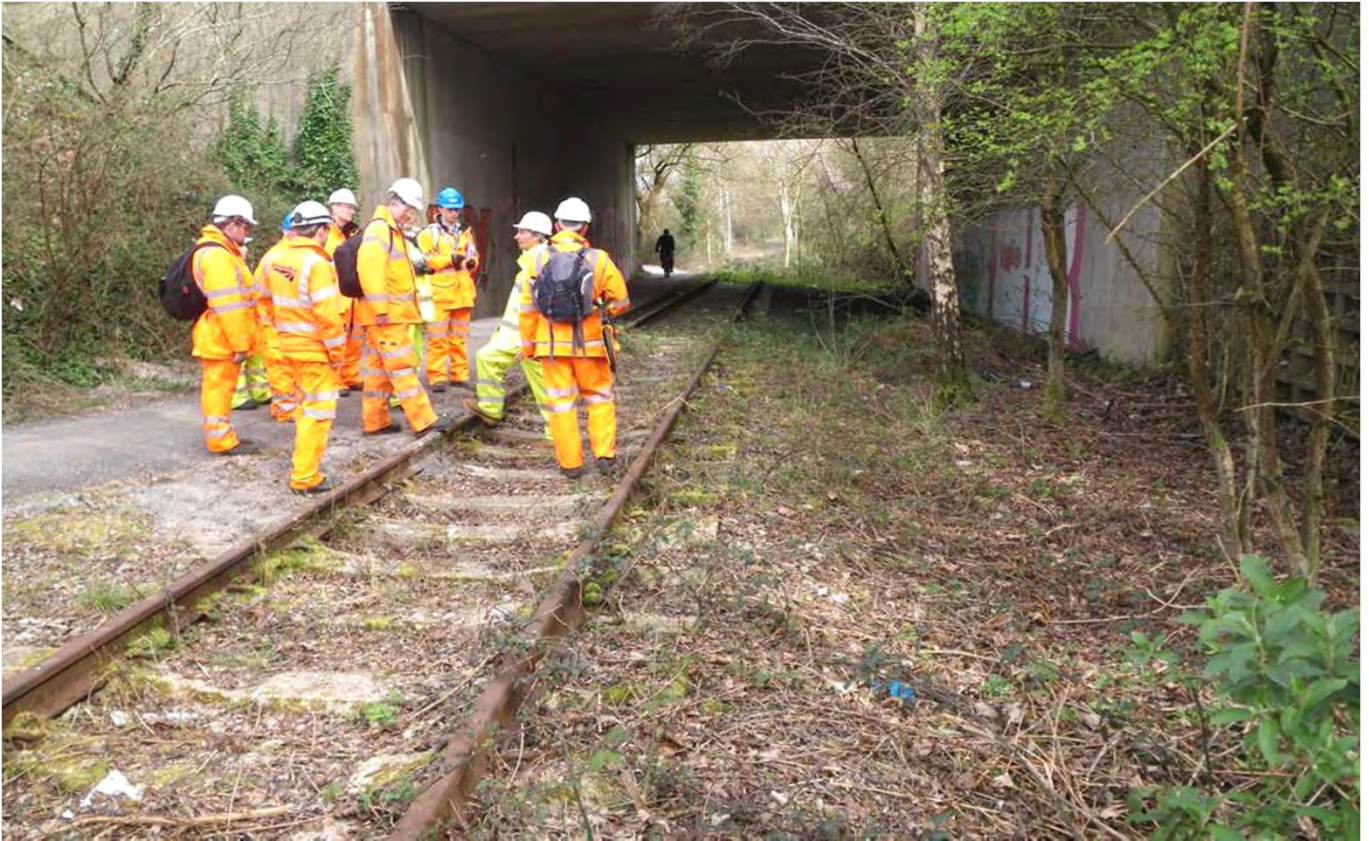
Photo 57. Facing Portbury Jcn at 127m 549y: Royal Portbury Dock Road Overbridge
