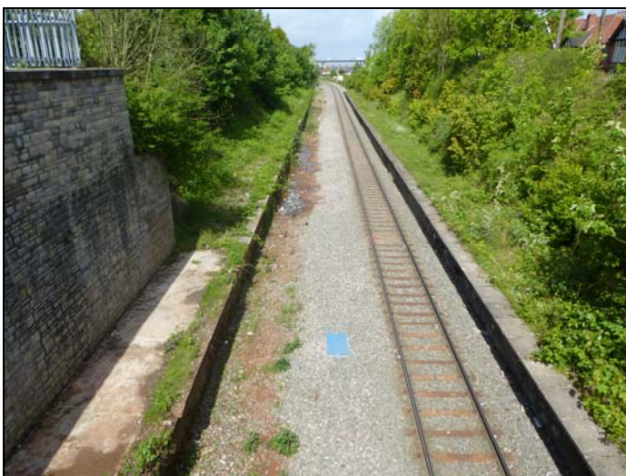
Pill Station platform – view from bridge towards Portbury
