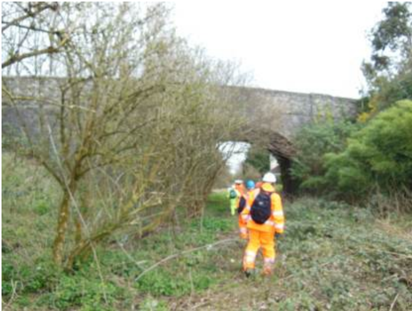
Figure 24– High mileage (West) side – overbridge adjacent to old Portbury Station
