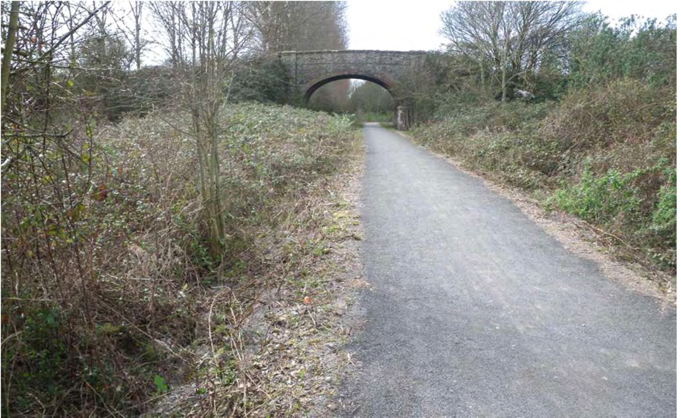
Photo 63. Facing Portishead at 127m 0y: Marsh Lane Overbridge
