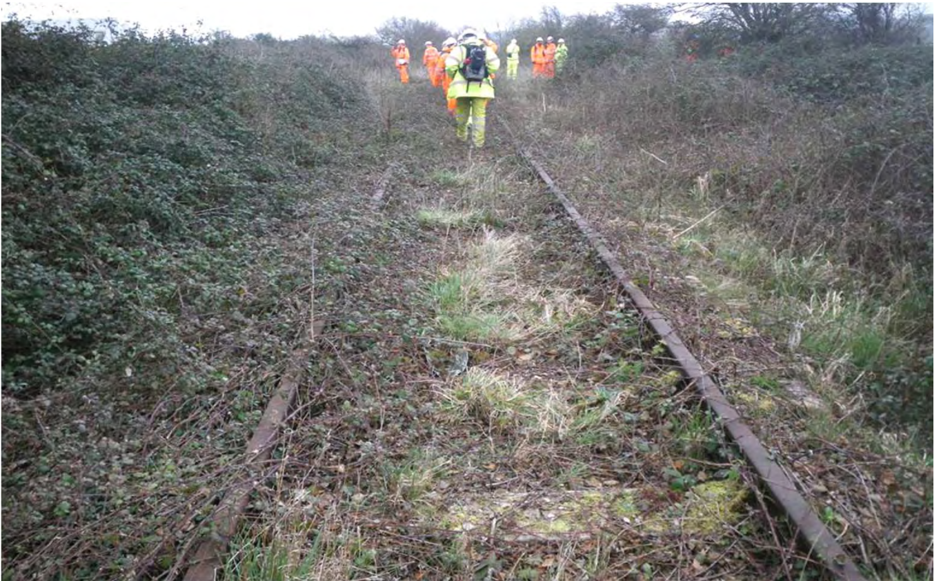
Photo 26. Facing Portbury Jcn at 128m 1054y
