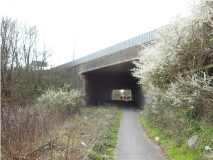
Figure 45 - Overbridge carrying M5 motorway: view from low mileage end
