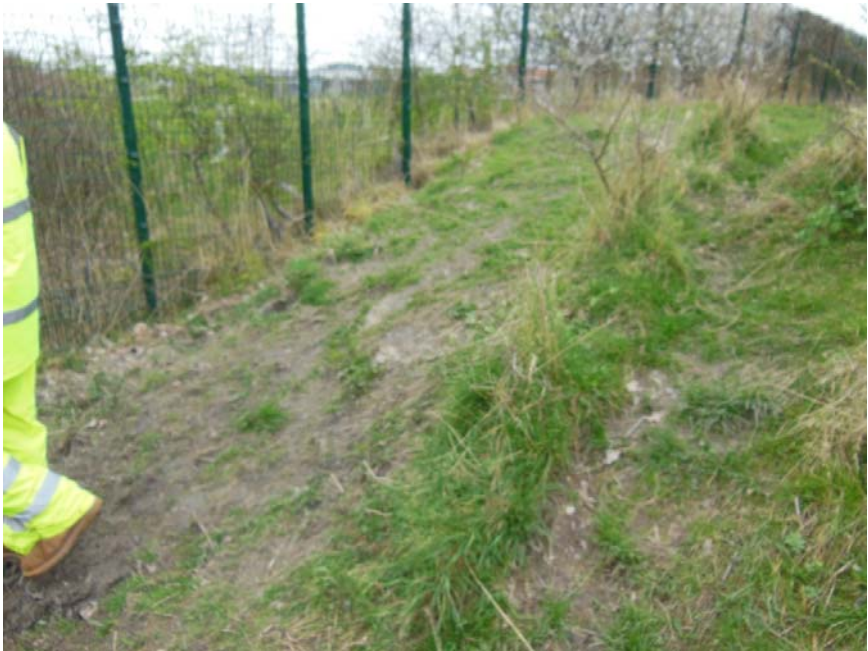
Figure 9 – View of embankment to the north of the line
