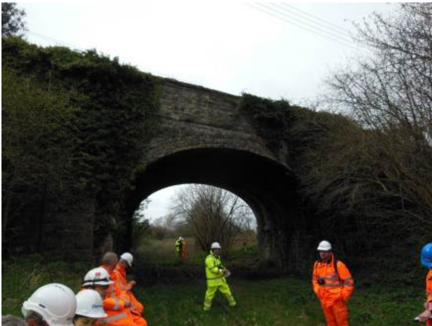
Figure 26- Low mileage (East) side – overbridge adjacent to old Portbury Station
