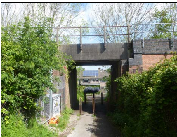
Avon Road Underbridge - location of proposed bridge widening
