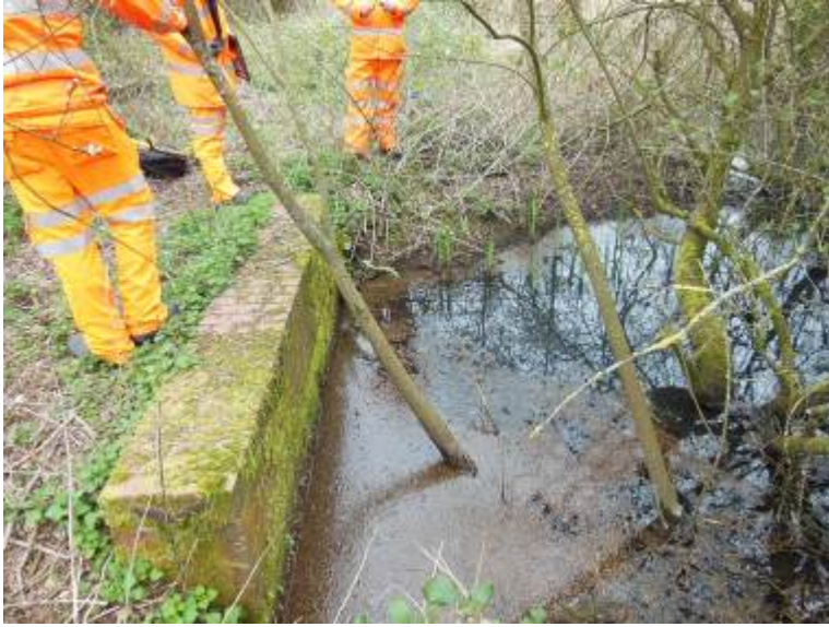
Figure 28 – Culvert A: view from South of the line
