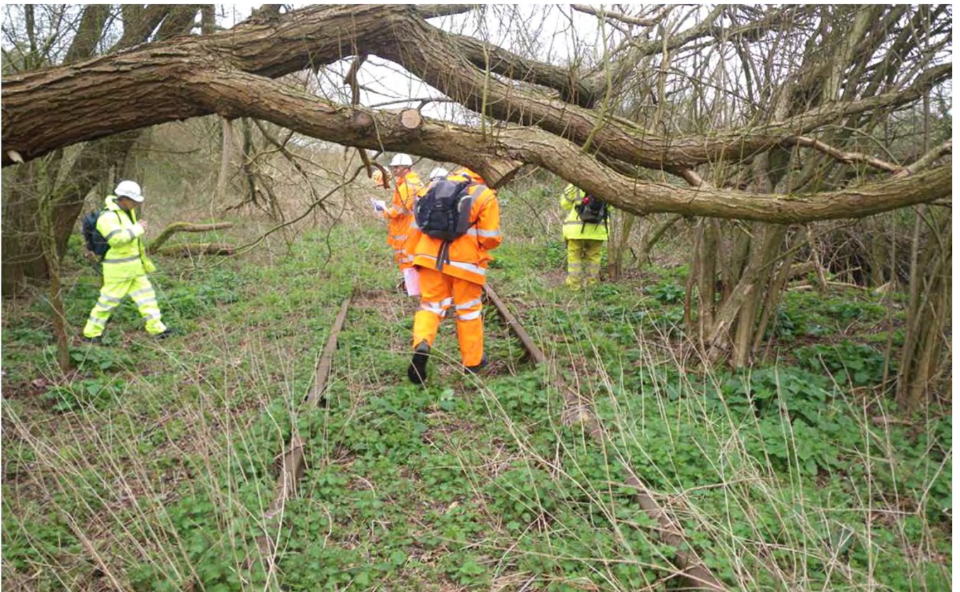
Photo 44. Facing Portbury Jcn at 127m 1548y
