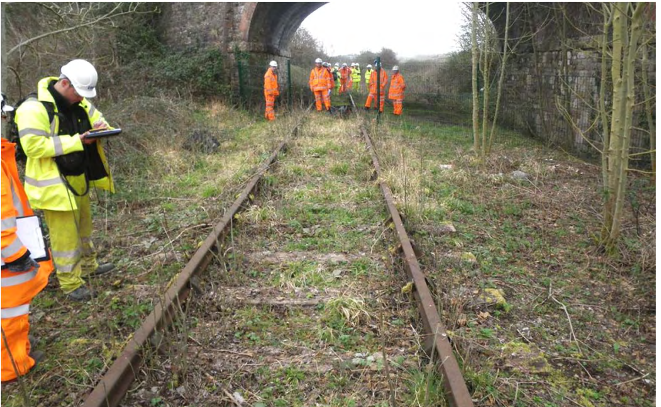
Photo 22. Facing Portbury Jcn at 128m 1239y: Sheepway Road Overbridge
