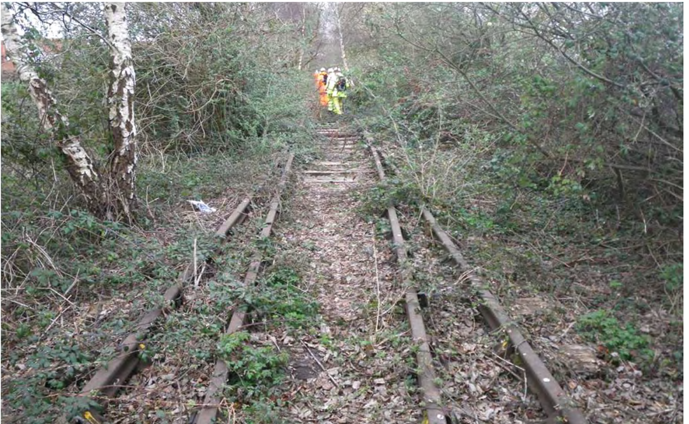
Photo 6. Facing Portbury Jcn at 129m 244y
