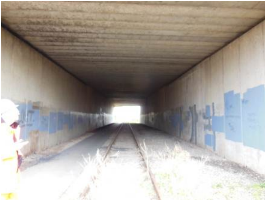
Figure 41 – View from high mileage end of underbridge – overbridge carrying M5 motorway
