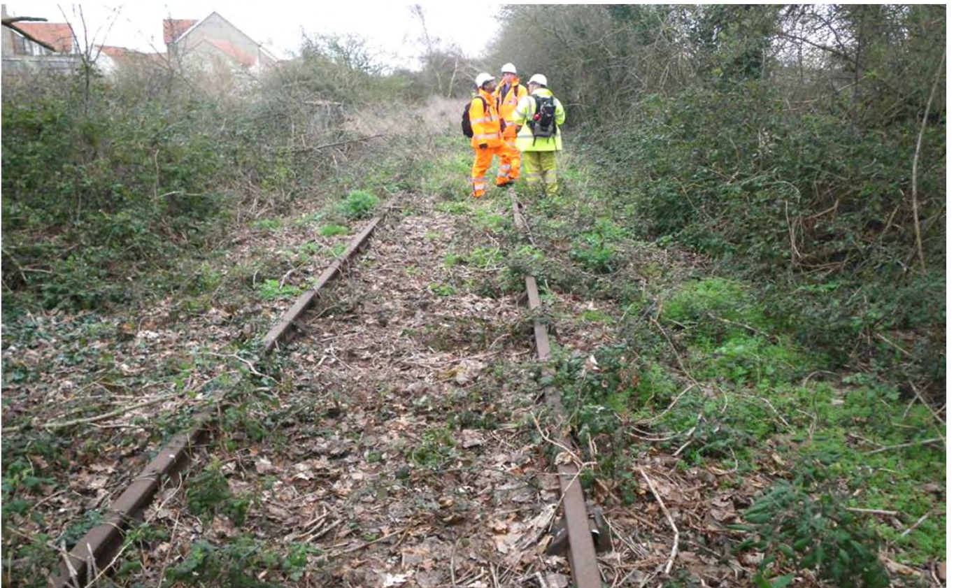
Photo 10. Facing Portbury Jcn at 129m 98y
