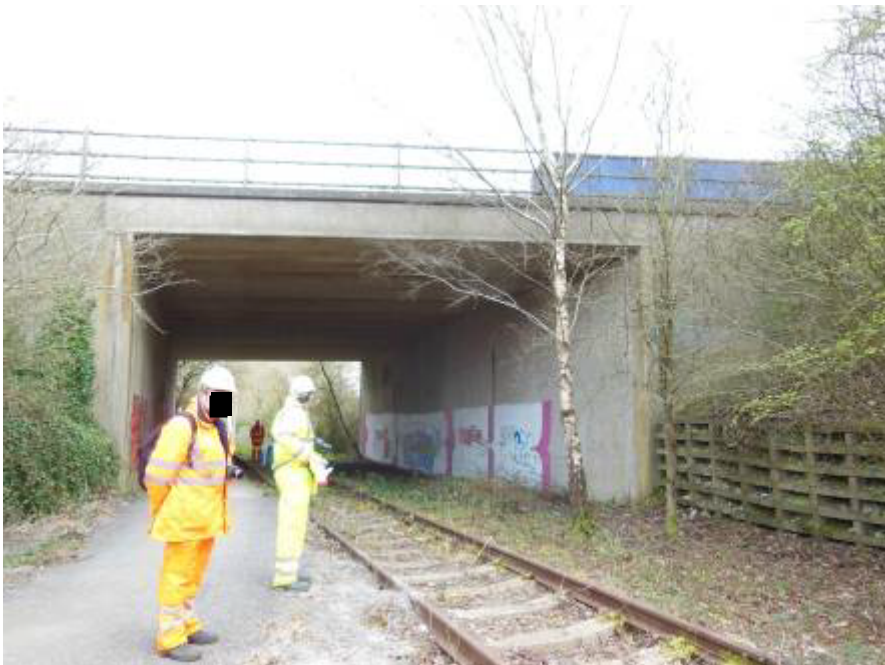
Figure 33 - Overbridge carrying Royal Portbury Docks Road
