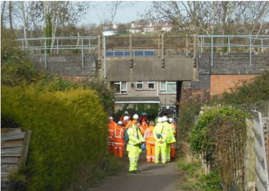
Figure 47 – South side of underbridge
