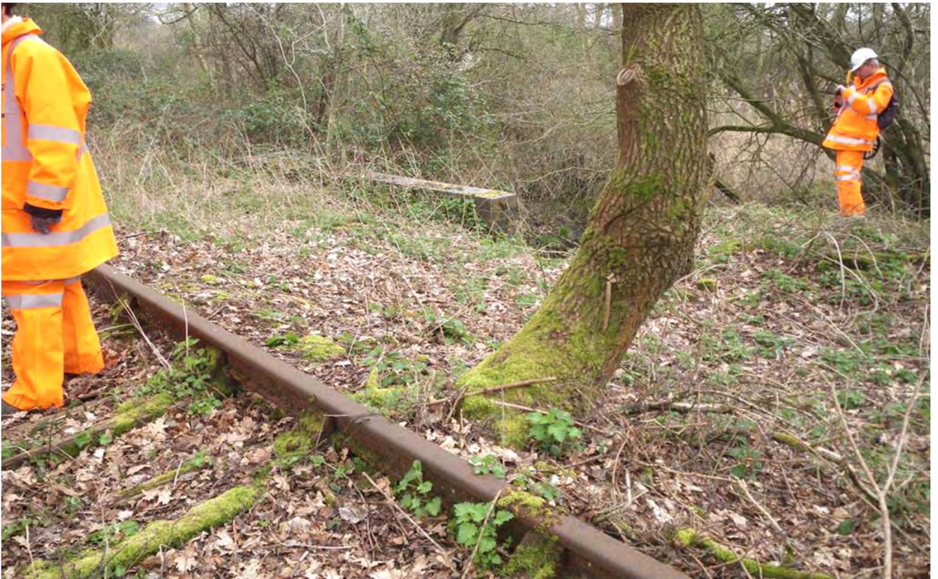
Photo 52. Facing Culvert at 127m 923y
