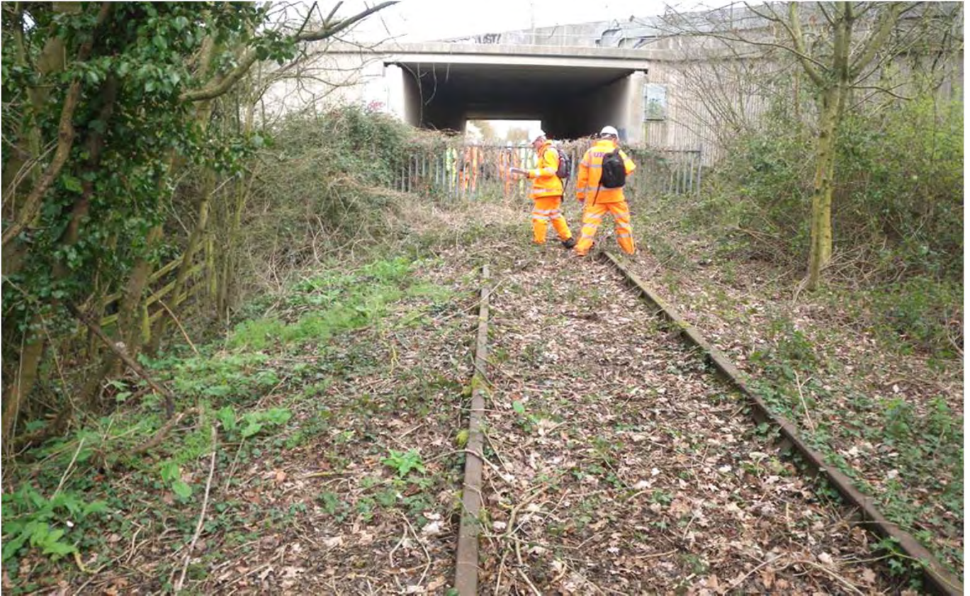
Photo 69. Facing Portbury Jcn at 126m 1385y: M5 Motorway Overbridge
