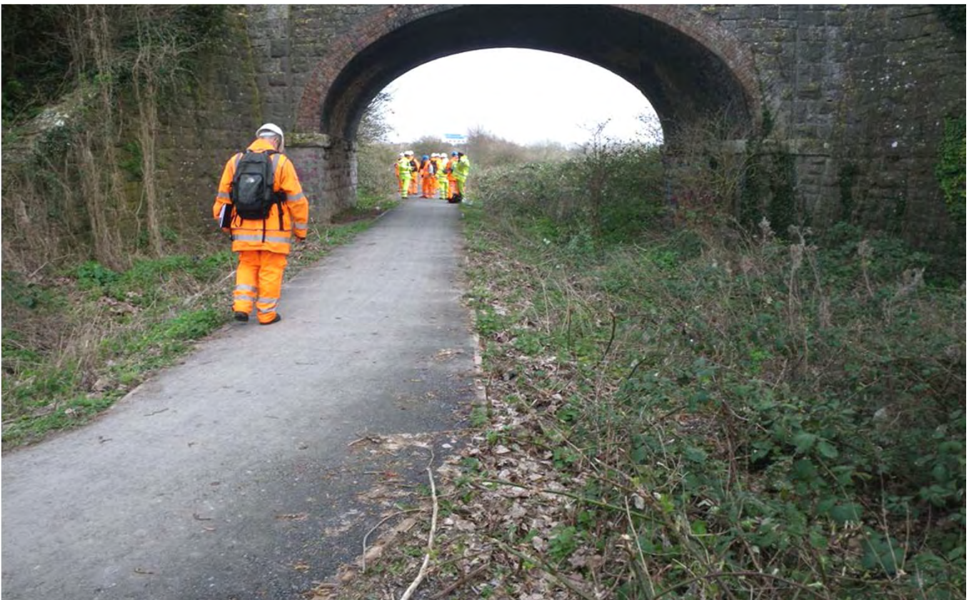
Photo 62. Facing Portbury Jcn at 127m 71y: Marsh Lane Overbridge
